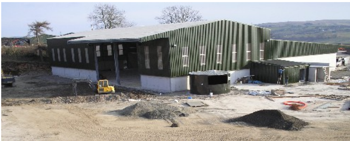
20,000 in-vessel compost facility at Bryn Quarry during construction.
